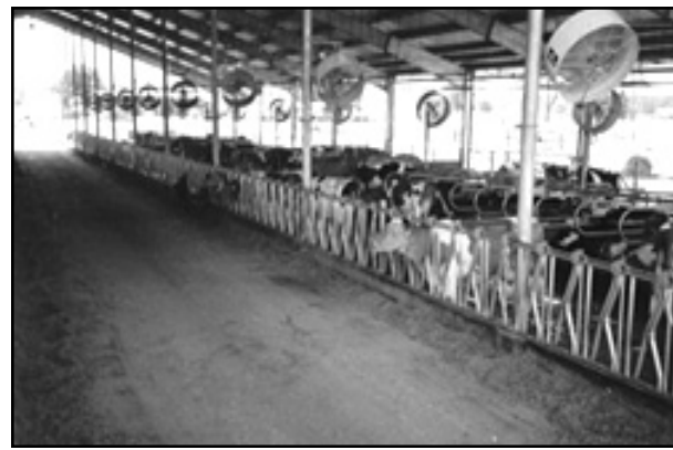
Figure 3 High speed horizontal fans to cool dairy cattle
