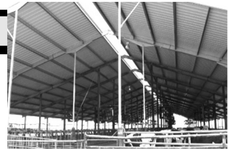
Figure 1 Naturally ventilated freestall barn
